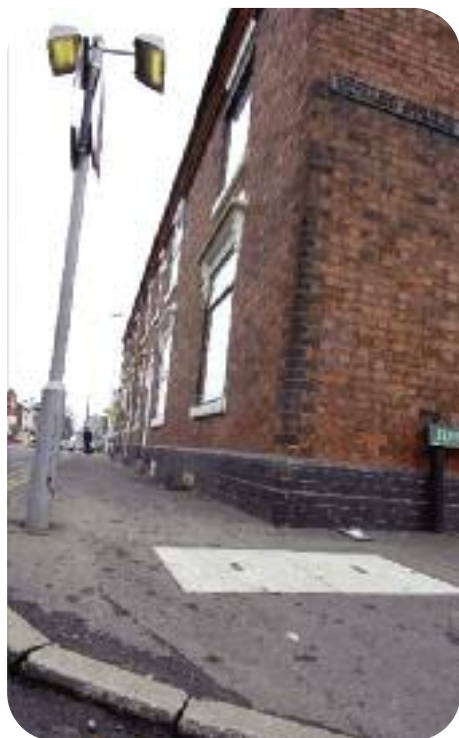
The junction of Dartmouth Street and Edward Street as it is now, which will benefit from the improvement work.
